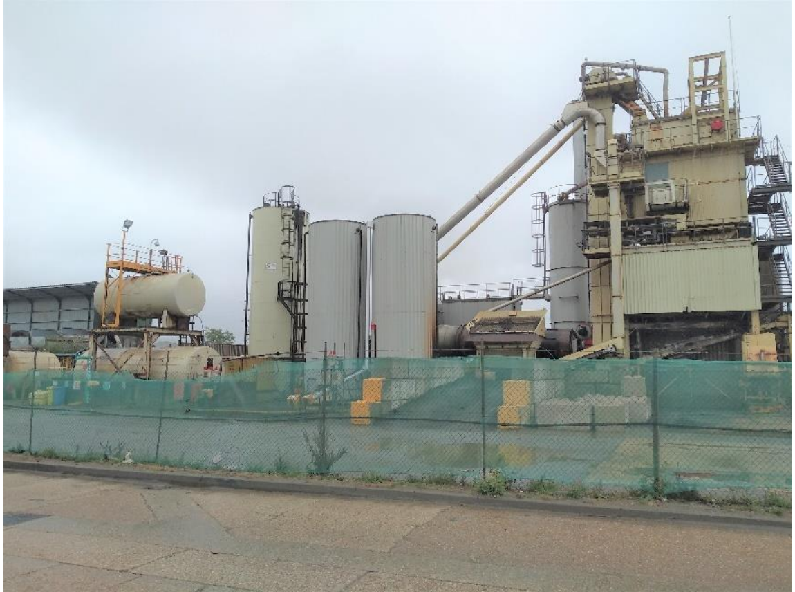
Figure 16: Oil and bitumen tanks outside the Tarmac process plant
