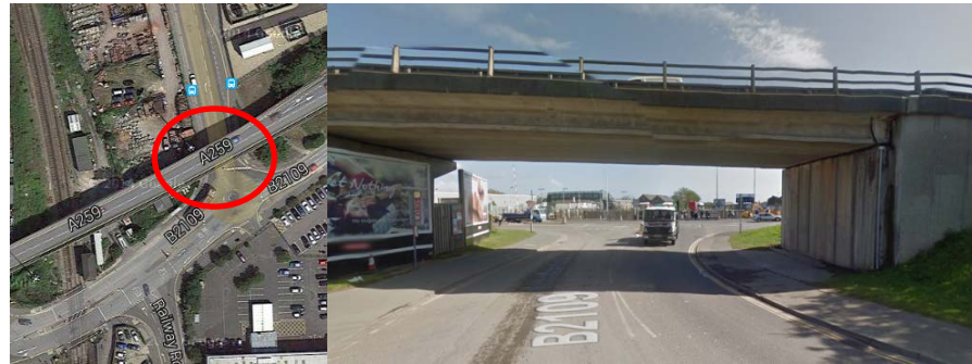
Figure 39: Under bridge crossing to access Drove Road
