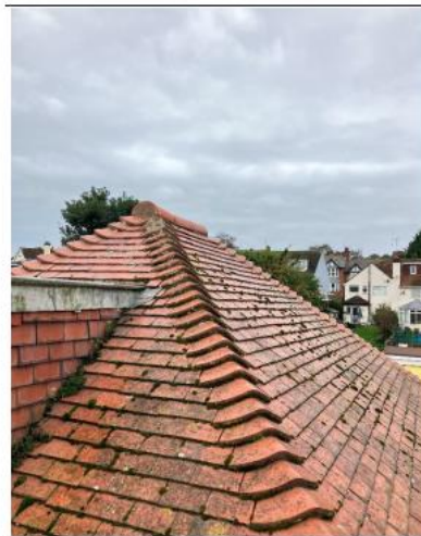
Roof 1- General view of pitched roof
