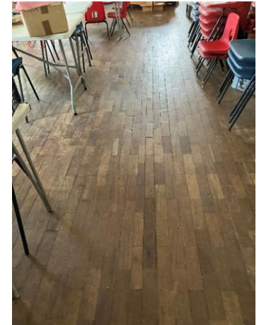
Main Hall 2- Warped Floor
