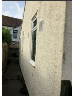
South Elevation 1 - General View
