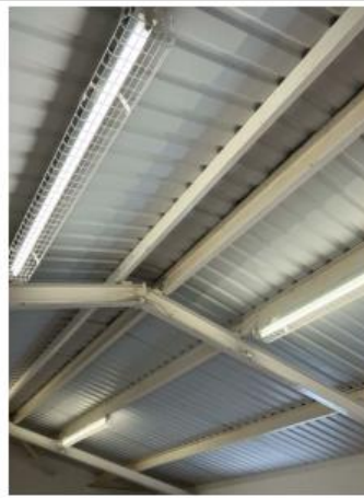
Hall 3 - Exposed Roof Structure
