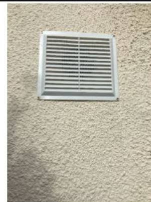
South Elevation 2 - Air Vents
