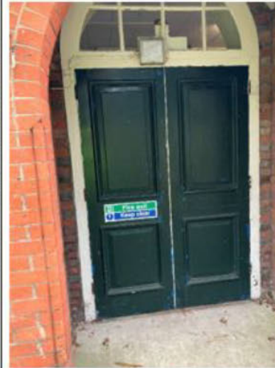
North Elevation 5 - Timber Fire Exit Doors
