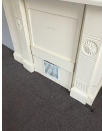
First Floor 2 – Closed Fire Place With Grill Vent
