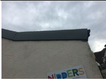
Fascias/Sofitts 1- North plastic fascia
