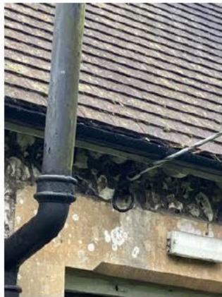
East Elevation 2 - Roof Drainage
