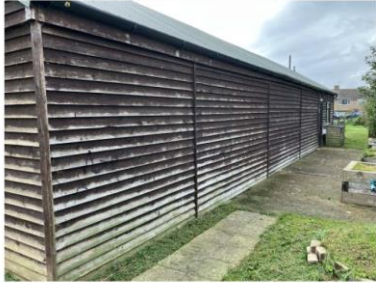
North Elevation 1- General View
