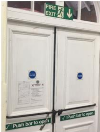
Ground Floor 6 – Internal Of Timber Fire Doors
