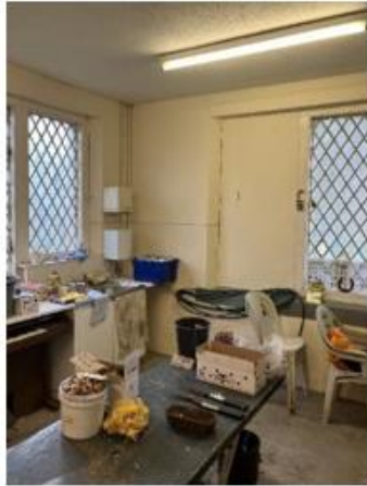
Morgue 1 – General View
