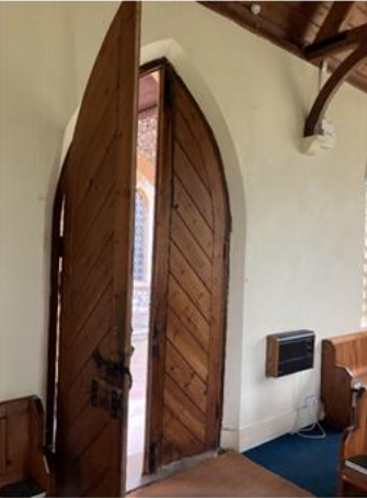
Chapel 3 – Timber Doors
