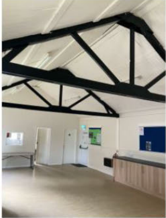
Hall 1 – General View
