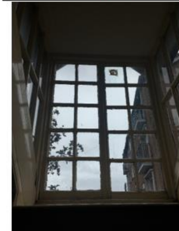
First Floor 7 – Dormer Window
