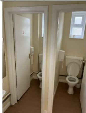
FT 1 - General View
