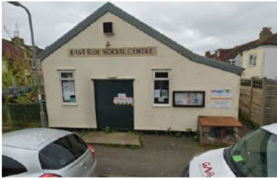
North Elevation 1 - General View
