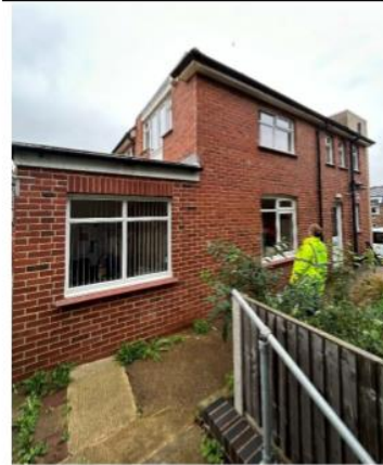
South Elevation 1 - General View
