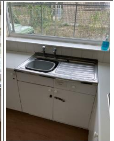
Kitchen 2 - General View
