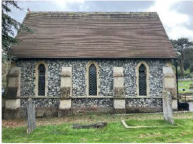
North Elevation 1 - General View
