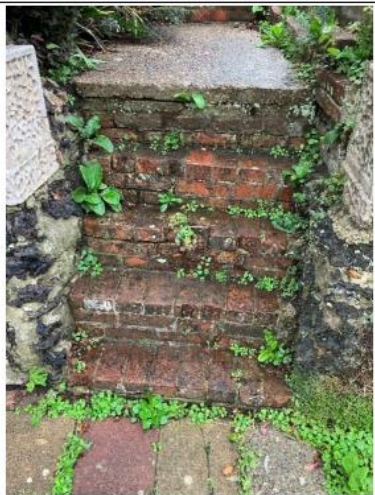
West Elevation 7 – Brick steps to raised area
