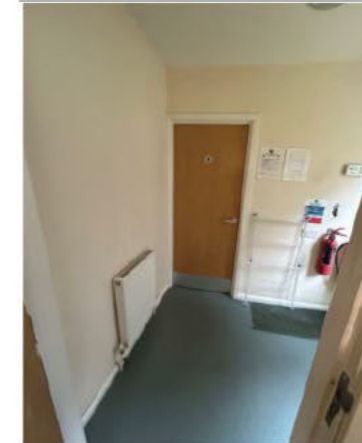
First Floor 6 - Corridor
