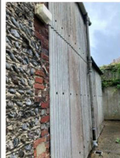
North Elevation 7 - Fibre Cement Panels
