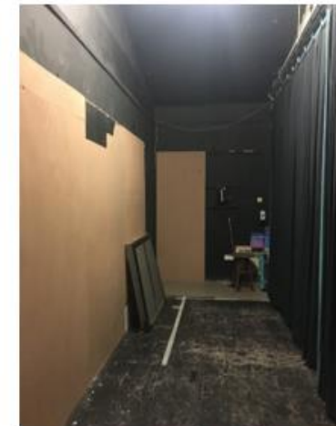
Ground Floor 3 - Area Behind Curtain
