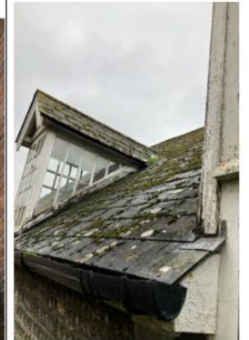
North Elevation 9 - Side Profile of Dormer Window
