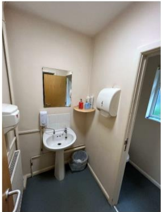
First Floor 8 – WC wash area
