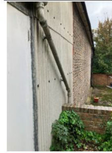
South Elevation 1- General View
