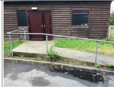
South Elevation 2- Concrete Ramp
