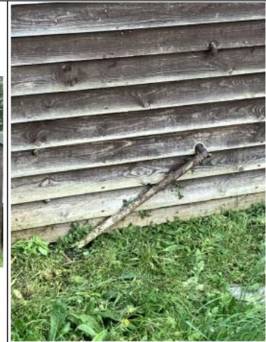
West Elevation 2- Drainage Pipes
