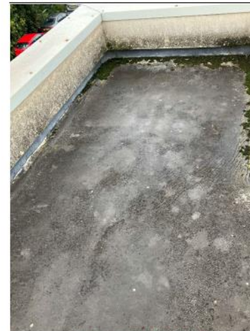
Roof 7 – Flat roof over lift shaft
