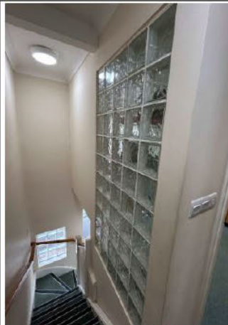
Staircase 2 - Staircase general view (descent)
