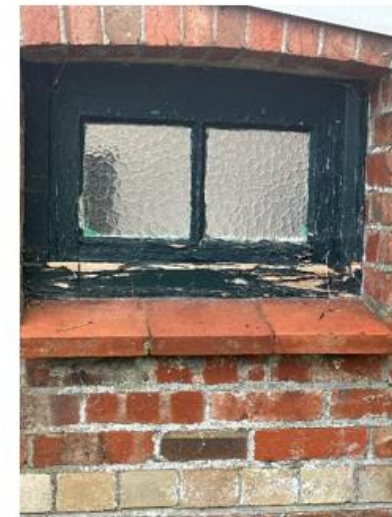
External Toilets 9 – Timber Window
