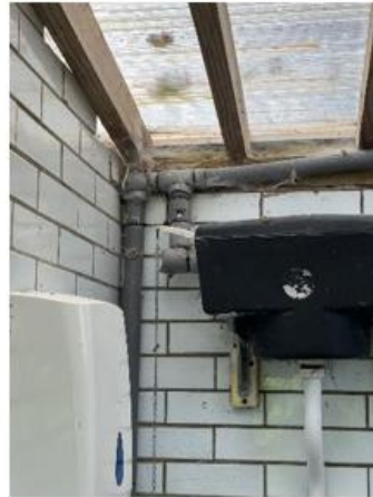
External Toilets 5 – General View
