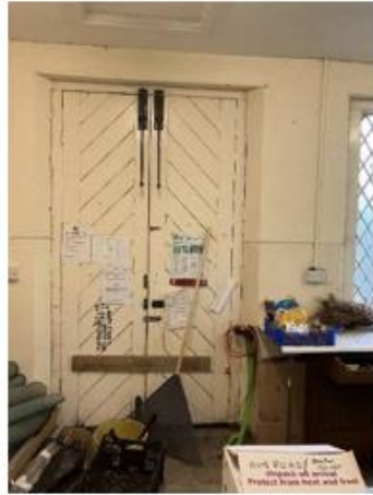
Morgue 2 – General View
