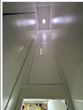
First Floor 11 – Internal lift shaft
