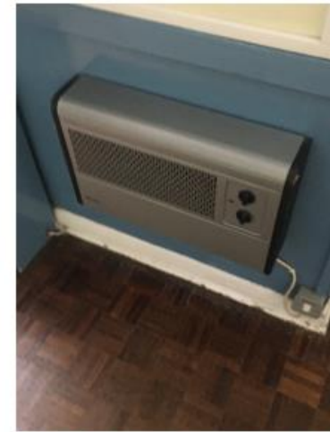
Ground Floor 1- Wood Flooring and Electric Heater
