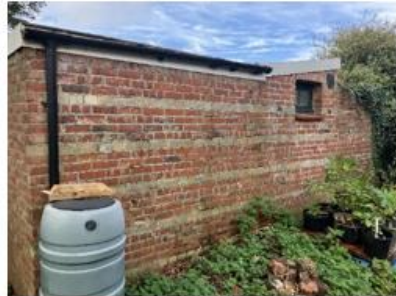
External Toilets 2 – Eastern Elevation
