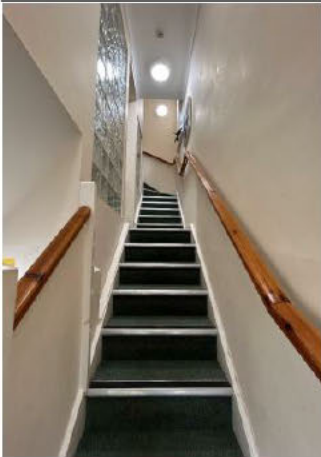
Staircase 1 - Staircase general view (ascent)
