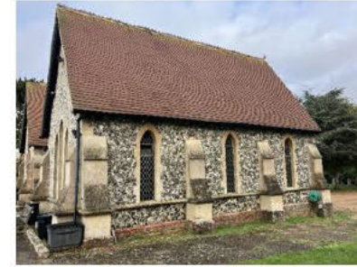
South Elevation 1 - General View
