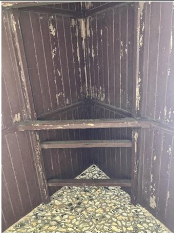
Central Archway 3 – Exposed Roof Structure
