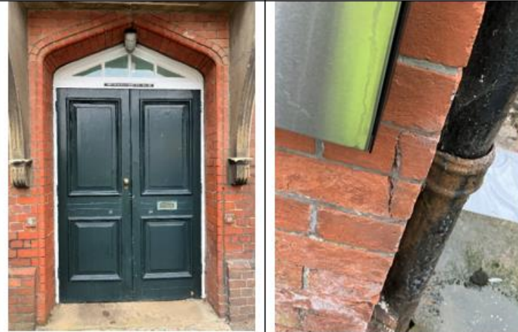
East Elevation 3 - Double Solid Timber Front Doors
