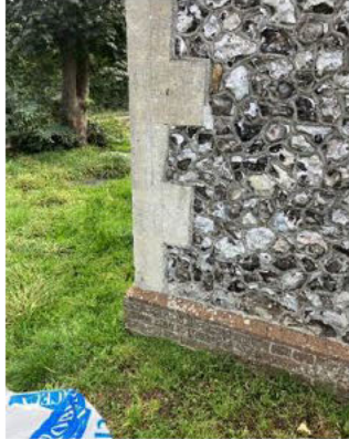
North Elevation 2 - Flint Wall on Masonry Plinth
