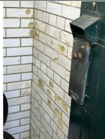
External Toilets 7 – Ceramic Wall Tiles
