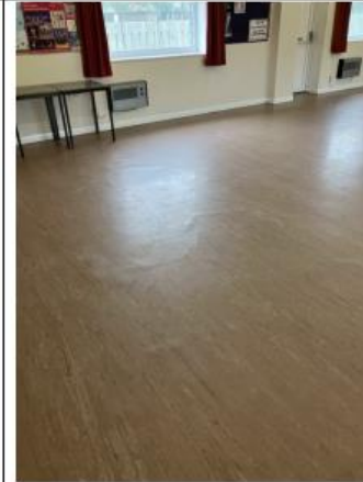
Hall 2 - Floor Finish
