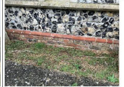
South Elevation 2 - Flint Wall with Masonry Plinth
