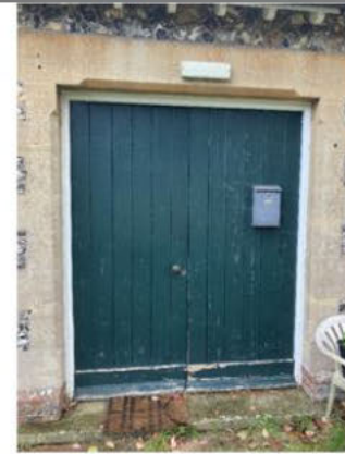
West Elevation 3 - Timber double-doors
