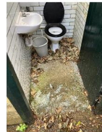
External Toilets 8 – Solid Floor
