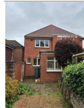
West Elevation 1 - General View from ground
