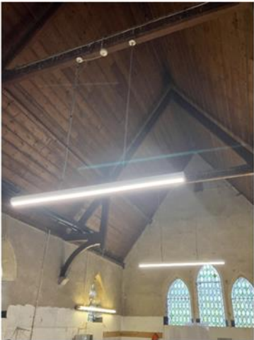
Workshop 5 – Exposed Roof Structure
