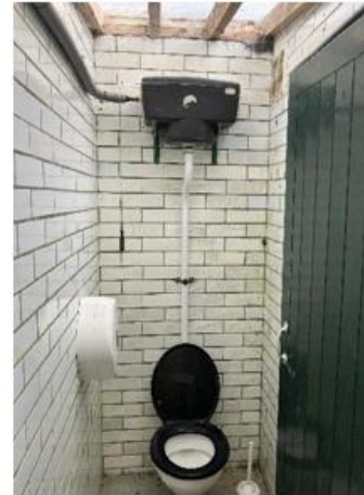
External Toilets 6 – General View
