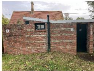
External Toilets 4 – Western Elevation
