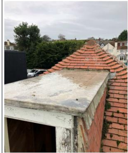
Roof 4 – Roof access through loft
