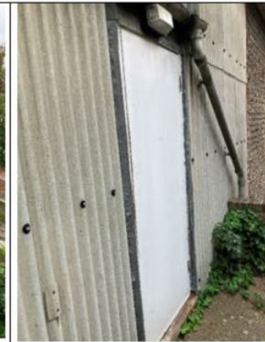
South Elevation 2- Timber Door
