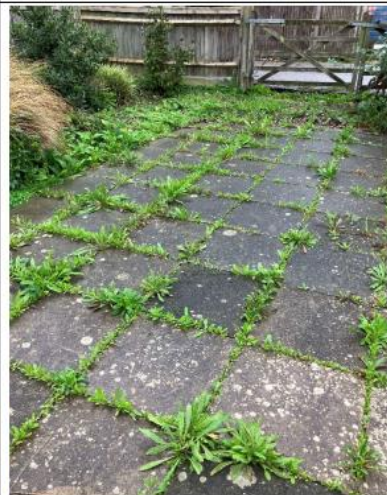
West Elevation 8 – Slabs
