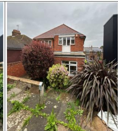
West Elevation 2 - General View from raised area
