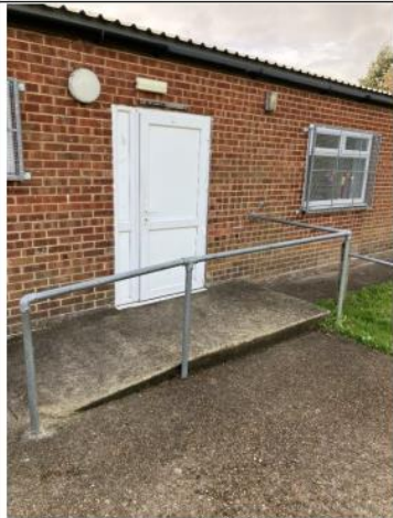
West Elevation 2 - UPVC Door/ Window
