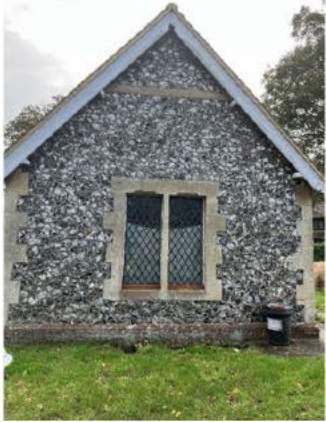
North Elevation 1 - General View
