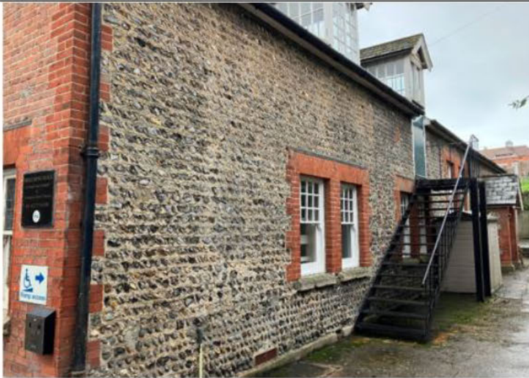
North Elevation 1- General View
