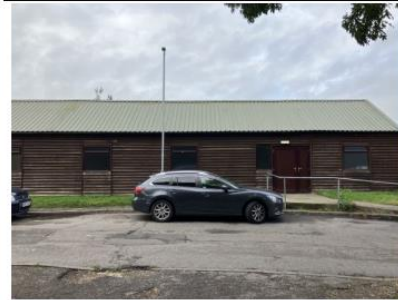
South Elevation 1- General View
