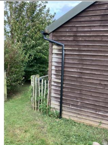
South Elevation 4 - Painted Timber Panels
