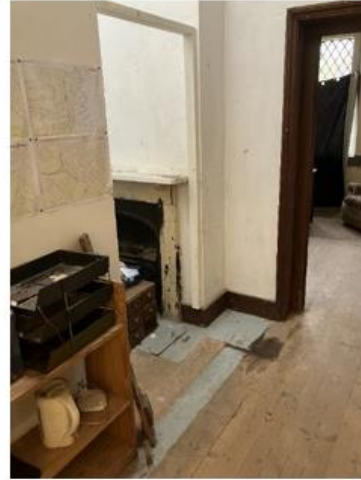
Sanitary Area 1 - General view
