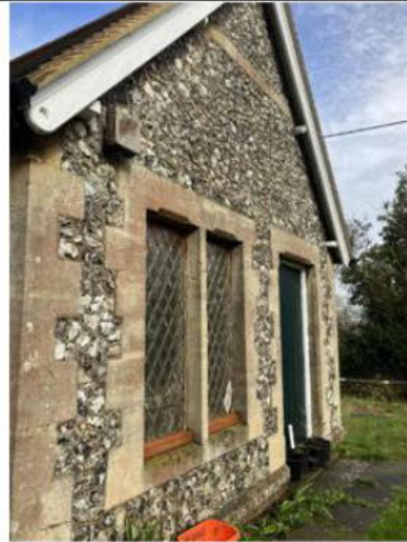
South Elevation 1 - General View
